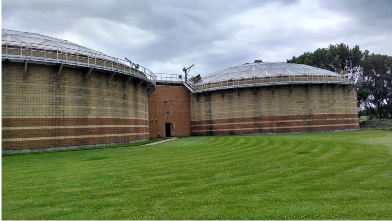
Anaerobic digesters (Stevens Point, WI)
