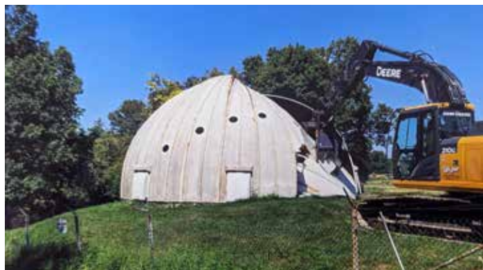
Eden's old trickling filter (top) was demolished and replaced with a new final clarifier (bottom).
