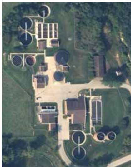
Overhead view of Platteville WRRF
