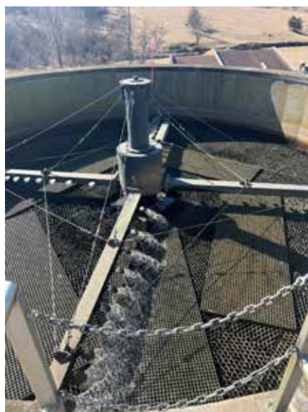
Top side view of the trickling filter at the City of Platteville WRRF
