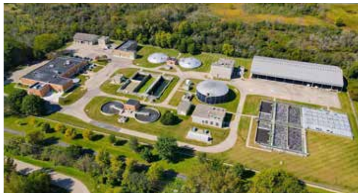
Aerial picture of the Fort Atkinson WWTP
