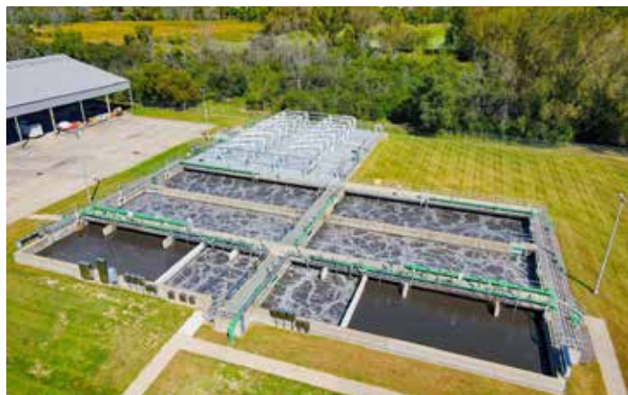
Aeration and digester
