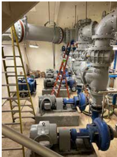
Five Fairbanks influent pumps with new forcemain center left, existing forcemain piping center right
