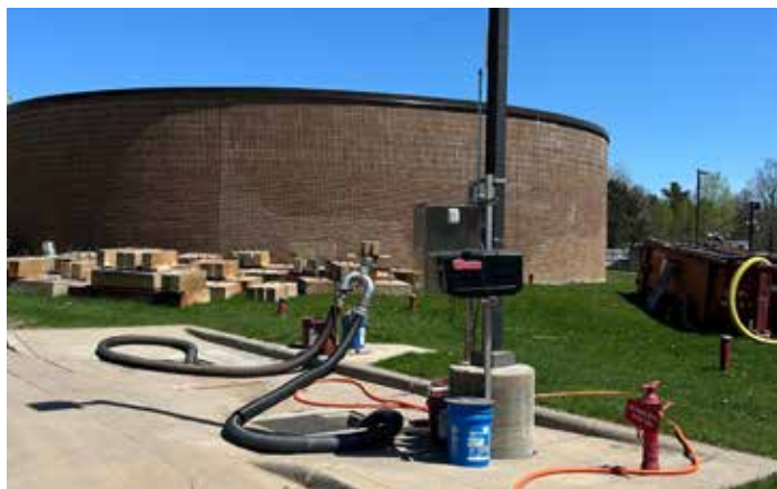
Septage hauler dump station in foreground, primary digester with crane supports in background
