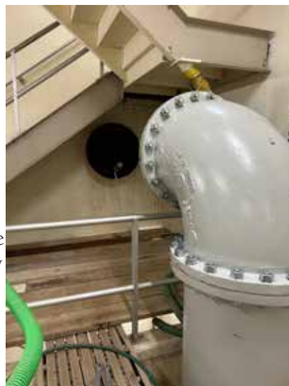
New forcemain entrance to pump house, waiting to be connected to pipe in dry well
