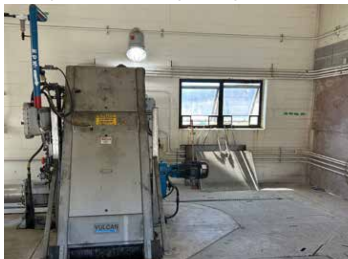
Existing Vulcan step bar screen, new Vulcan step bar screen going in on the right side of picture
