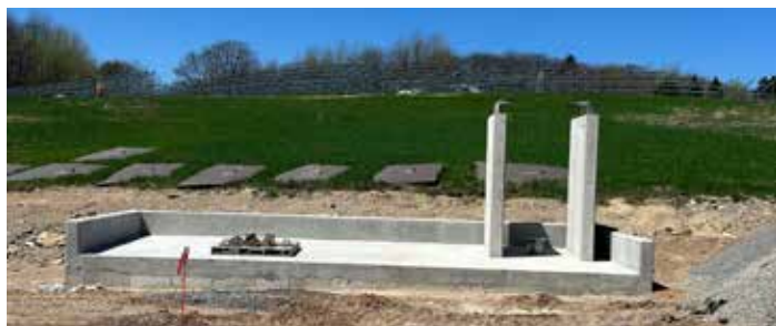
New waste gas burner pad in foreground, primary digester cover sections mid-ground, solar array in background
