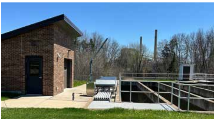
UV building on left, UV in use in middle, old chlorine contact tank on right
