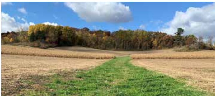
A Grassed Waterway in La Crosse County, installed with MDV funding, prevents gully erosion from delivering sediment and nutrients to nearby surface waters.
