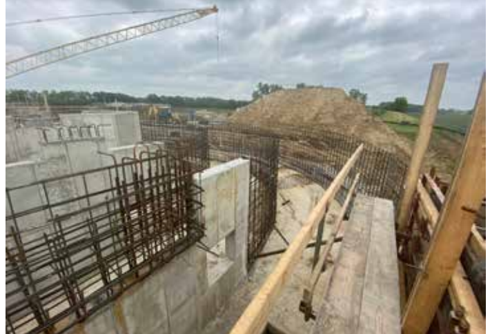
Oxidation ditch construction
