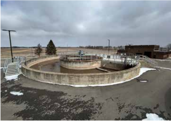
Digester sludge storage
